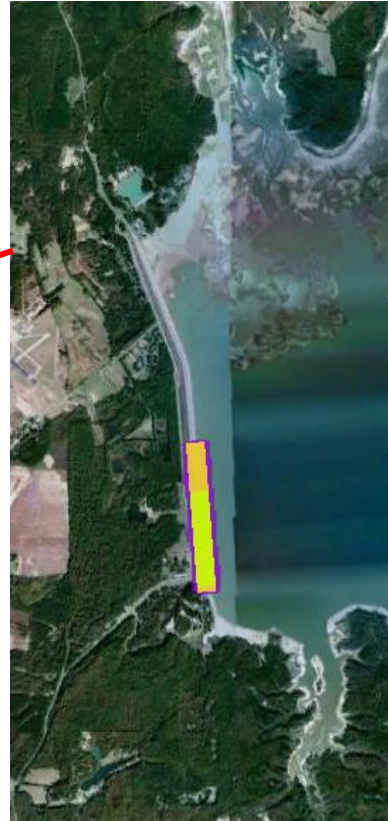
The dam is defined too short. The water leaks over the undefined part of the crest.
