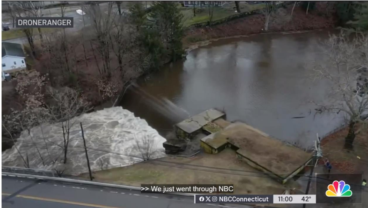
All eyes are on a dam that sprung a leak and led to hundreds of people being told to leave their homes in eastern Connecticut. That evacuation order has since been lifted.
