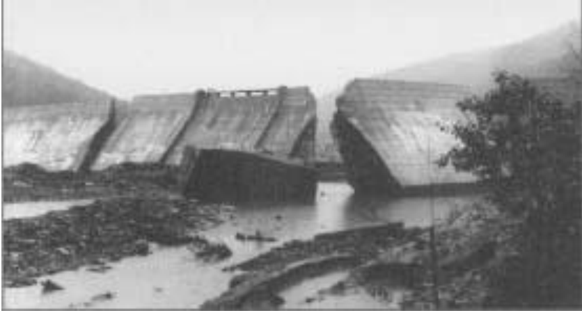
Remnants of the Austin, Pennsylvania, dam after its failure on September 30, 1911.
