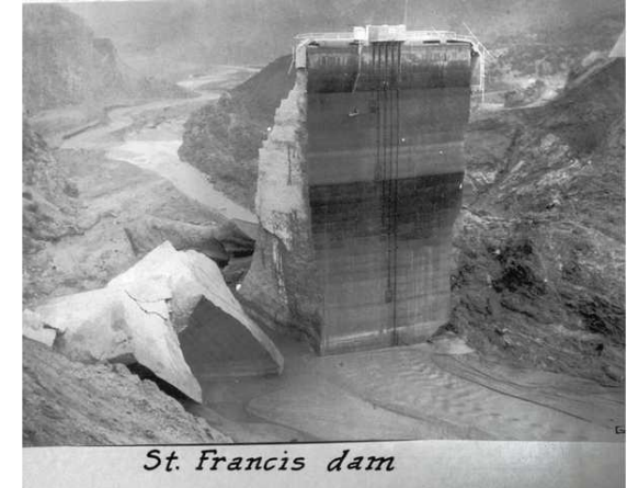
On March 12, 1928, St. Francis Dam gives way in Los Angeles, failed killing over 500 people. The St. Francis Dam was a curved concrete gravity dam, built to create a large regulating and storage reservoir as part of the Los Angeles Aqueduct.
