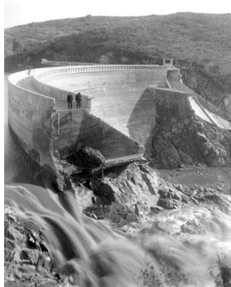
Sweetwater Dam failure of 1916
