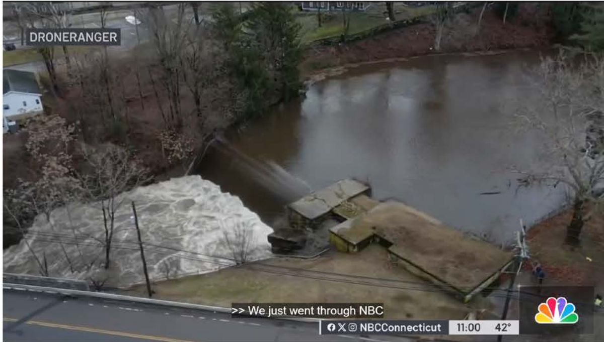
All eyes are on a dam that sprung a leak and led to hundreds of people being told to leave their homes in eastern Connecticut. That evacuation order has since been lifted.
